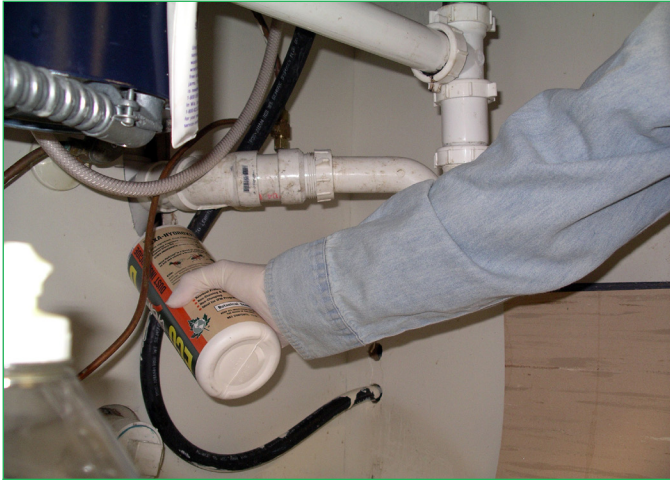
Figure 11. Applying dust to a wall void where plumbing pipes enter the wall.
